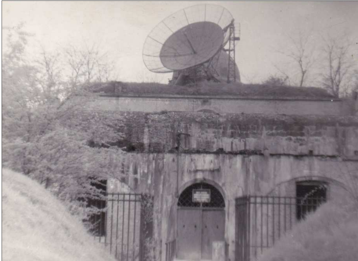
Figure 1: Fort Skala, an old Austrian fort, was the first radio astronomical observatory of Jagiellonian University. On the roof is the 7-m antenna that later was used for solar monitoring (courtesy: Jagiellonian University Archive; henceforth JUA).
