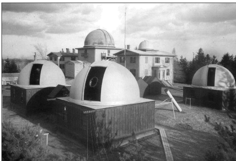
Fig. 7a: Harvard College Observatory in 1887, looking southeast from the cottage used as a dark-room. In the foreground are: 0.32-m and 0.25-m photographic telescopes in the leftmost dome; the 0.20-m Bache astrograph in transit shed; 0.70-m f/5 reflector in the middle dome; 0.38-m reflector mounted in open; 0.28-m f/14 Clark photographic refractor in third dome, at right. From First Annual Report of the Henry Draper Memorial project , published in 1877.
