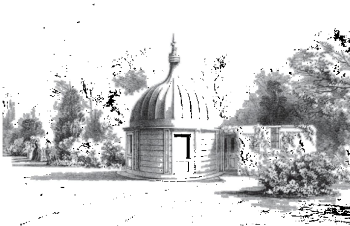
Figure 2. The South Villa Observatory, comprising the tapered dome of the equatorial room, and the adjoining transit room. (Courtesy the Library of the Royal Astronomical Society)
