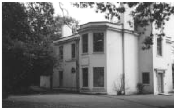
Figure 3. Broadgate House as it appears today
