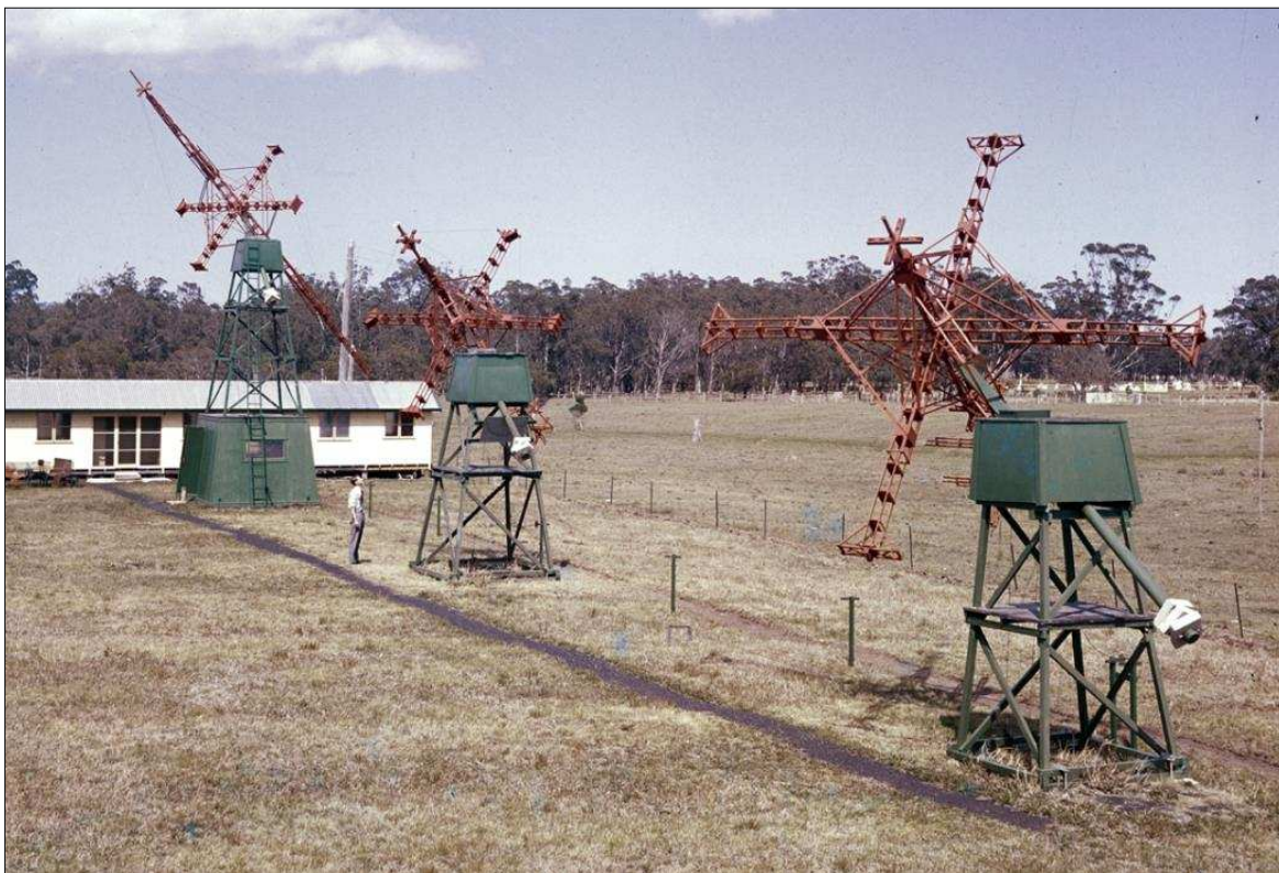
Figure 23: The Dapto field station, showing the three crossed-rhombic antennas and associated buildings (RAIA 12429-1).
