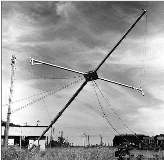
Figure 22: The rhombic aerial of the world's first radio spectrograph, at RP's Penrith field station (RAIA).
