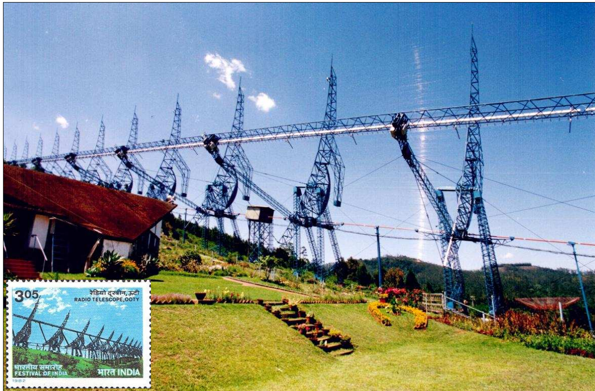
Figure 47: Another view of the Ooty Radio Telescope; reflections of sunlight by 1,100 stainless steel wires are seen on the right. The inset bottom left shows an Indian stamp featuring the ORT (courtesy: TIFR Archives).
