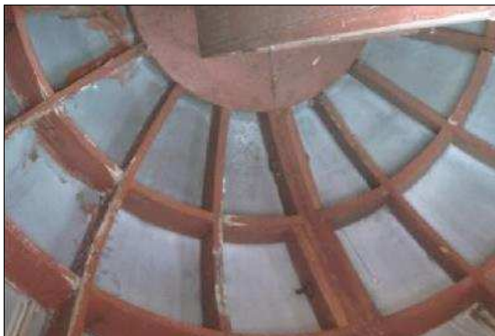
Figure 11: Internal framing of the Lyttelton time ball (courtesy: Bruce Carr).
