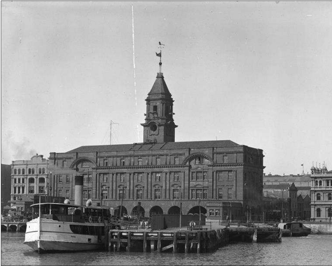
Figure 16: The Auckland Ferry Building on 8 April 1913 showing the time ball on the mast (courtesy: Auckland Libraries, Sir George Grey Special Collections, 1-W1555).
