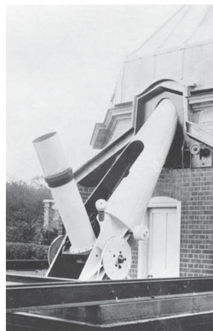
Figure 11. The Cambridge Sheepshanks 32cm f/18.5 telescope seems to have been the inspiration for Strachan’s telescope. It was used at public open nights, between 1898 and 1959. Royal Astronomical Society/Science Photo Library.
